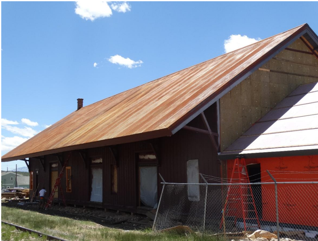
Freight Depot, Leadville. Prior to rehabilitation.
